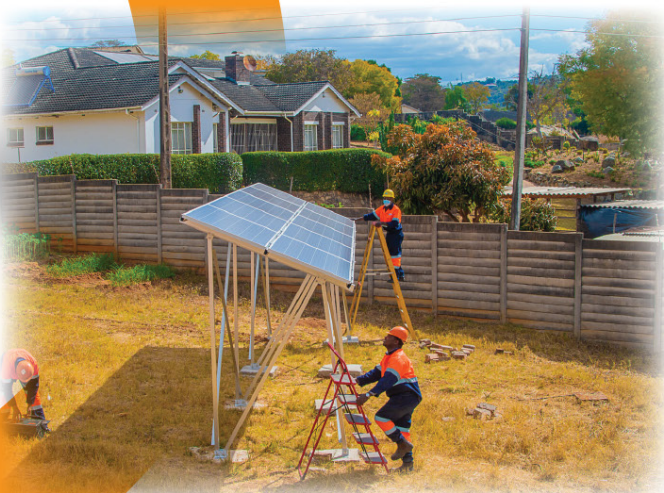
Borehole Solar System Installation
